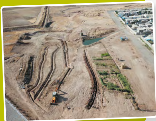
Drainage ground work, Gawilan Camp, N. Iraq
